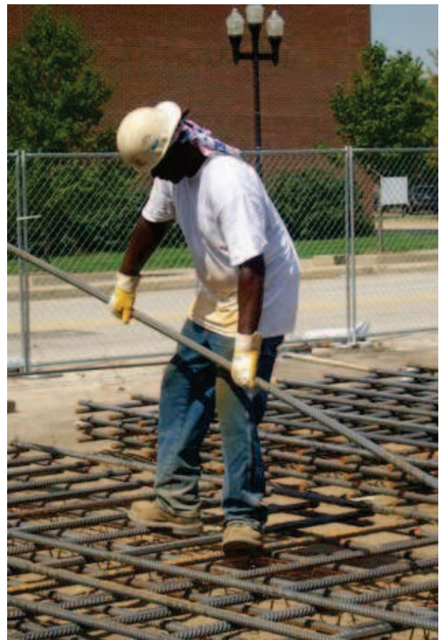
Iron Worker Preparing Reinforcement Mat for Footing
