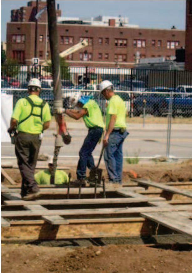
Pouring Concrete Footing along Monroe Street
