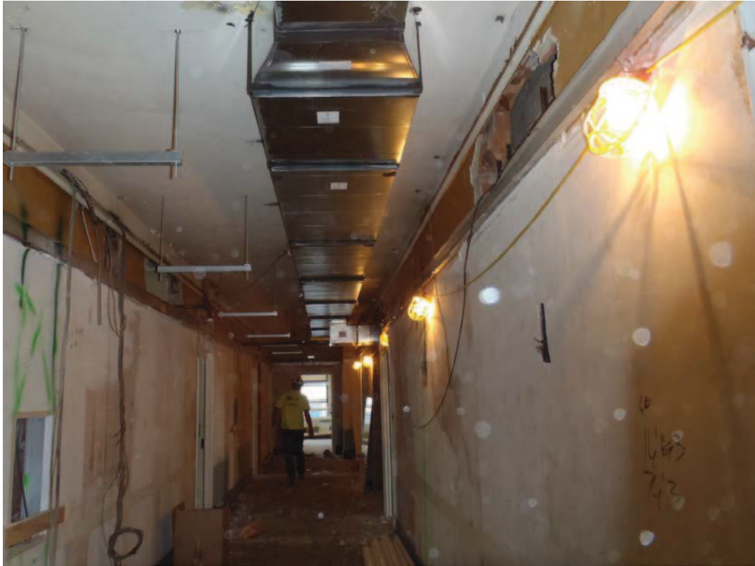
Ductwork installation on twelfth floor
