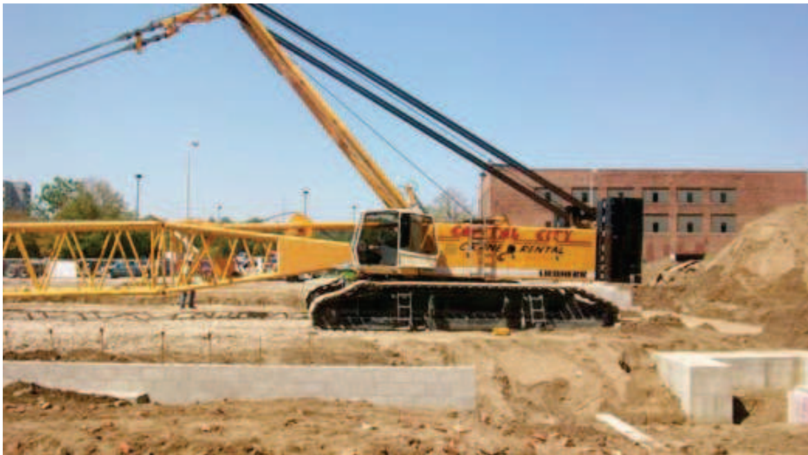
300 Ton crane being assembled
