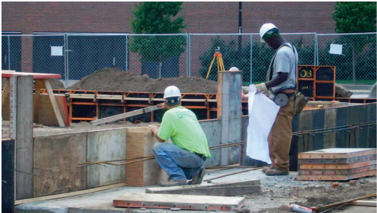
Forming of Foundation Stem Wall
