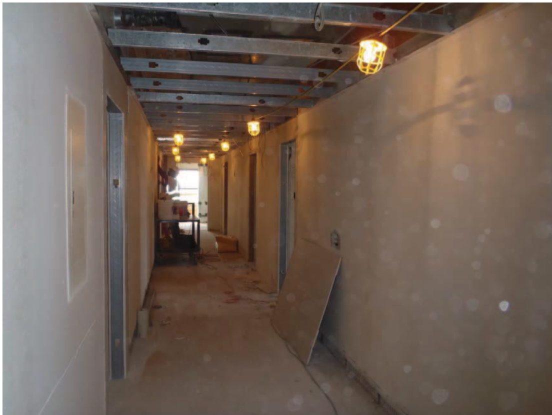
Drywall installation on ninth floor
