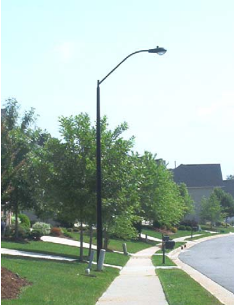
Figure 21. This residential street has cobra-head street lanterns, similar to those that are located along high-speed highways. These lanterns are out of scale with the pedestrian and are spaced so widely that the next lantern cannot be seen from here.
