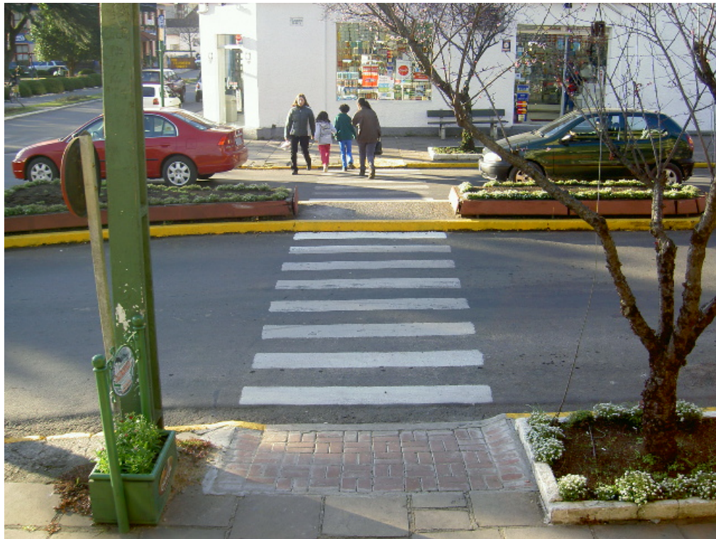
Figure 20. A landscaped island serves as a pedestrian refuge. A clearly marked crosswalk is located one car length from the intersection.
