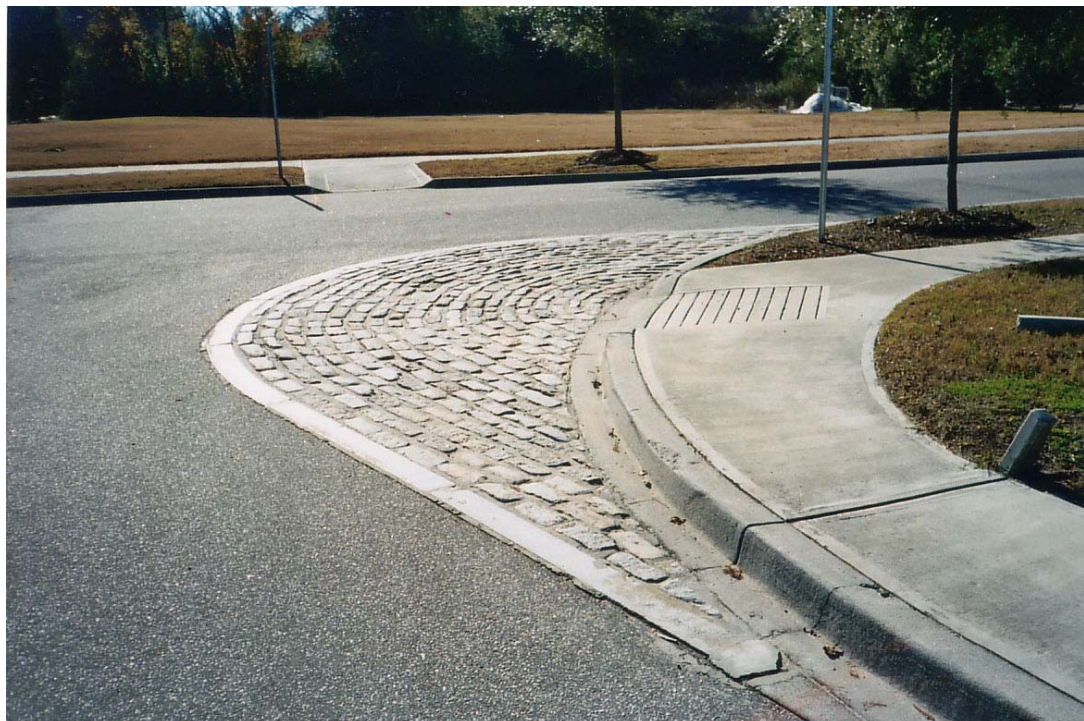
Figure 15. This creative solution, found at l'on Village in Mt. Pleasant, South Carolina, has a double curb line, one for car drivers, and the other for the occasional passage of emergency vehicles. Drivers generally follow the tighter curb radius because the zone of cobblestones does not appear to be part of the automobile realm but rather a part of the pedestrian realm.
