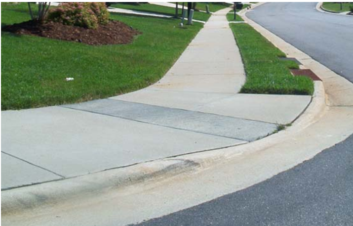
Figure 12. This curb radius is so large that a car can make the turn without braking at all. Few drivers slow down at these types of intersections.
