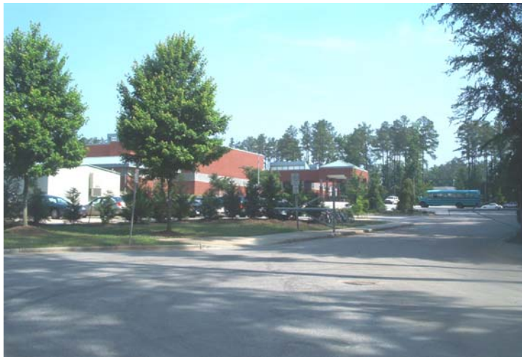
Figure 18. This large curb cut in front of Durant Road Middle School does not have a clearly marked crosswalk.
