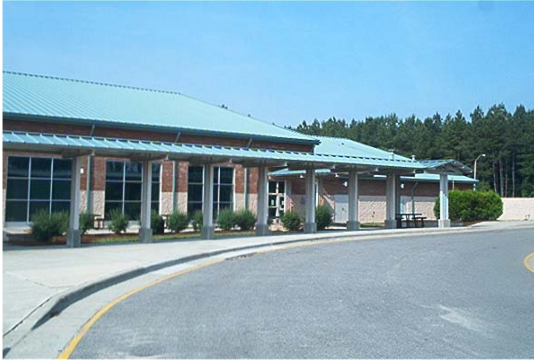
Figure 36. Wildwood Forest Elementary. Covered walkways and waiting areas are a welcome refuge from intense sun and rain.
