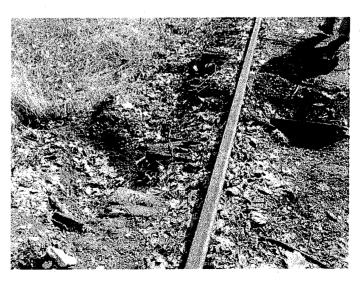
North side of railroad tracks – Brush in the ditch is restricting proper drainage. Brush should be removed.
