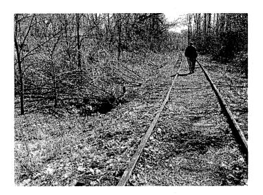
North side of railroad tracks – Brush in the ditch is restricting proper drainage. Brush should be removed.
