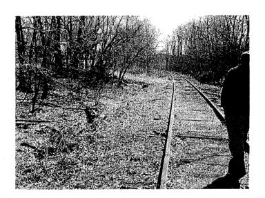
North side of railroad tracks – Erosion has occurred near the culvert. Gravel should be replaced and the bank properly shaped and stabilized.
