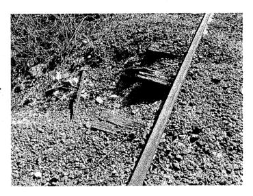
North side of railroad tracks -- Erosion has occurred under end of railroad ties. Additional gravel should be placed under the ties and the area stabilized to prevent further erosion.
