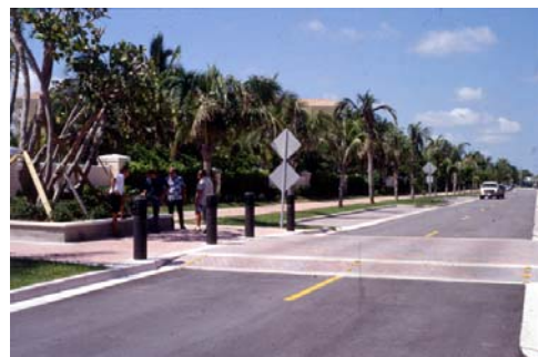
Figure 6.1: Raised Pedestrian Crossing
