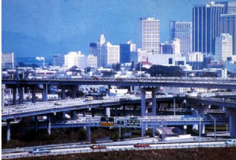
Figure 8.4: I-95 and I-395 through the Overtown Neighborhood, Miami
