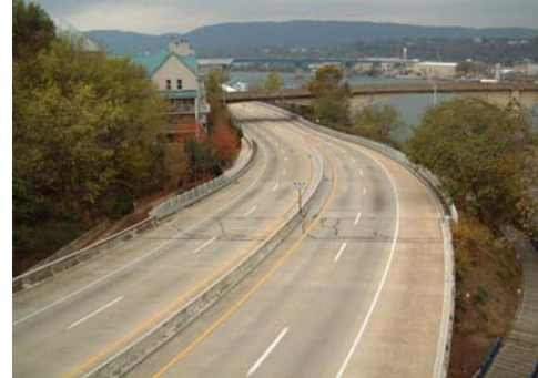
Figure 8.15: Waterfront Highway cuts off City.
