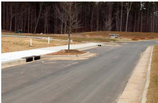
Figure 6.18: Narrowings without Valley Gutter
